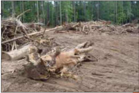
Grubbing of trees, shrubs and roots
