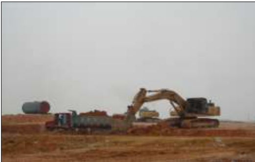
Excavator heaping up top soil
